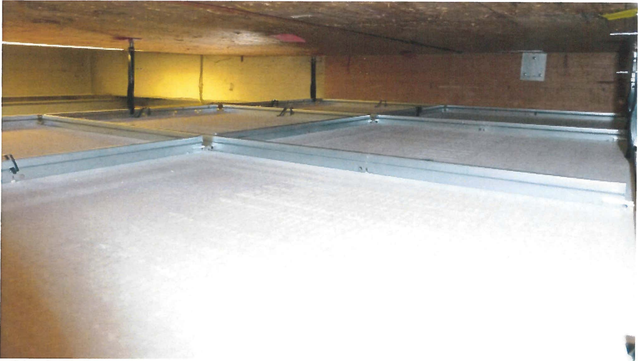
Picture 2 Detail: substructure „PLAZA S 24 Unity U 3“
