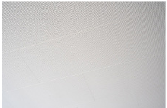
1200X600 INSTALLED IN STRAIGHT EDGE DESIGN
